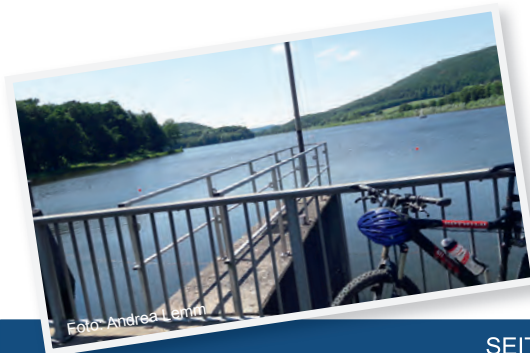
Staumauer Schieder See
